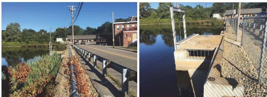
Upstream wall and trash racks after repairs
