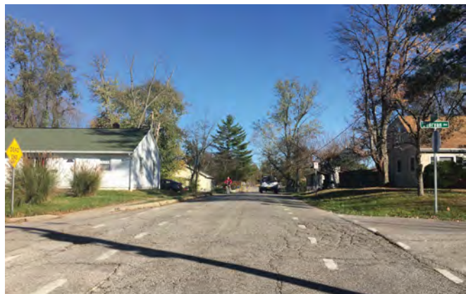
Sidewalks with curbs can be expensive to implement. For low-traffic residential streets, simple pavement marking can indicate safe shoulders to travel on.
